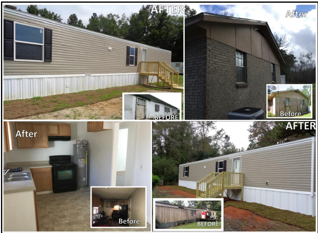
The South Carolina Disaster Recovery Office has repaired or replaced over 300 homes in Williamsburg County. Above is just some of their work.
