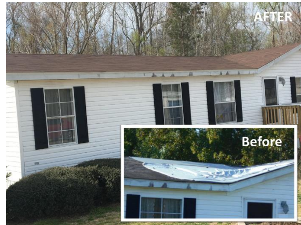
Before and After of Mrs. Burch's new roof.
