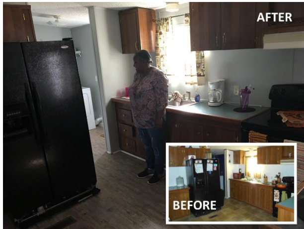
Mrs. Burch standing in her newly repaired kitchen.
